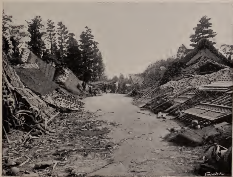
RESULTS OF THE EARTHQUAKE
